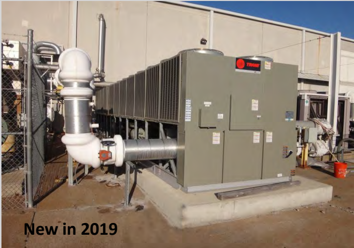
View of UNUSED Trane Chiller for Plant Air & Process
