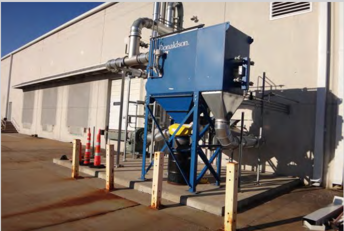
View of Torit Dust Collector
