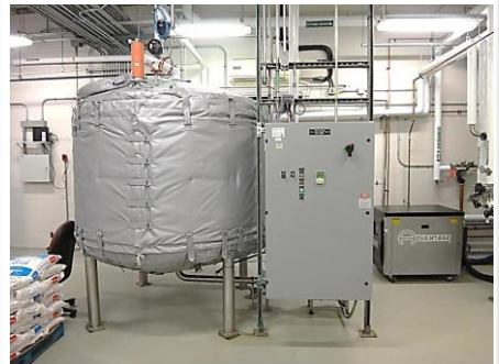
Evoqua (Siemens) USP Water System capable of 7 GPM. Includes 5000 Liter Stainless Steel Holding Tank, Aquafine DI Unit, and related. Turnkey System, in Operation
